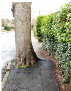
Problem: 40cm gap (No 18)
